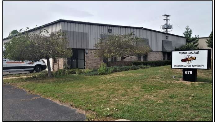
New NOTA sign installed
